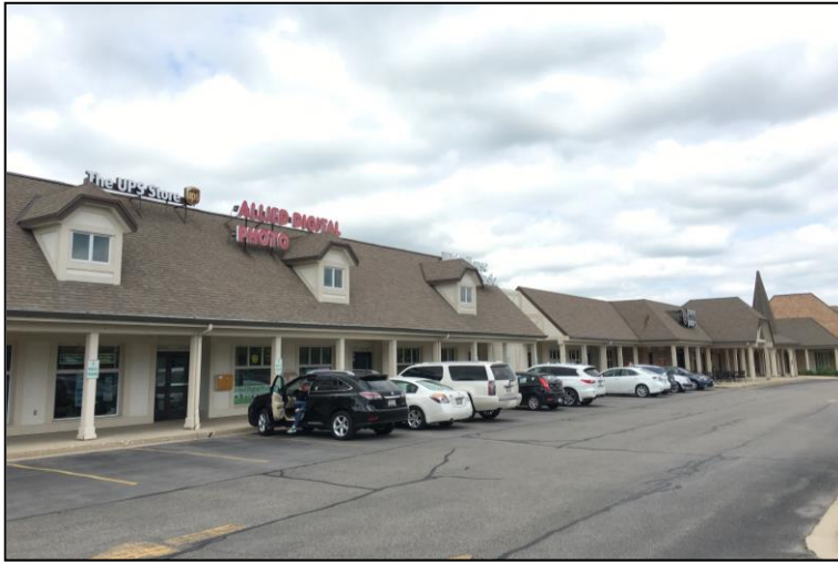
Phase I – Inline tenants
