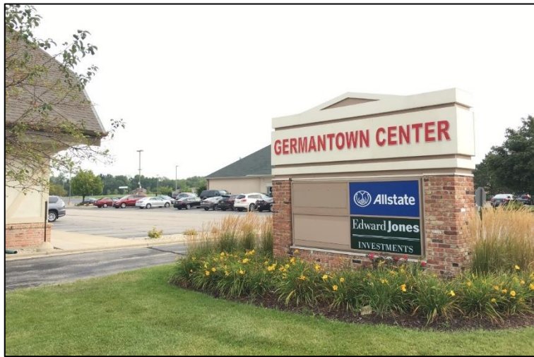
Phase II - Signage
