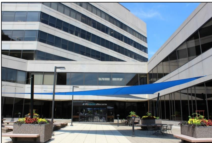
Main Building Entrance (Floor 2)
